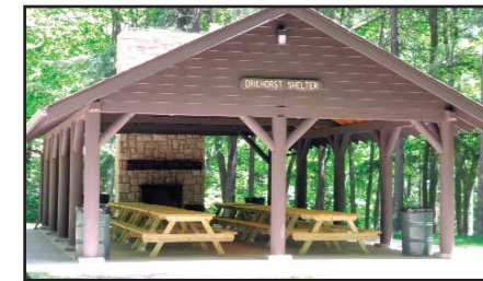
The mantle over the fireplace was constructed using a wood column from the old shelter, symbolically connecting the old to the new.
